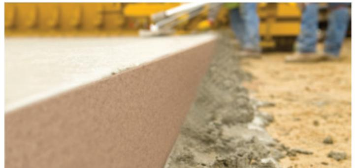
*Image above shows pre-formed strip adhered to adjacent slab to form the longitudinal construction joint.*
