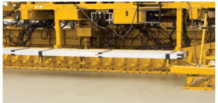
*Slip formed continuous concrete pavement uses the SPANDEX System as an integral part of the paving operation for both construction and contraction joints.*
